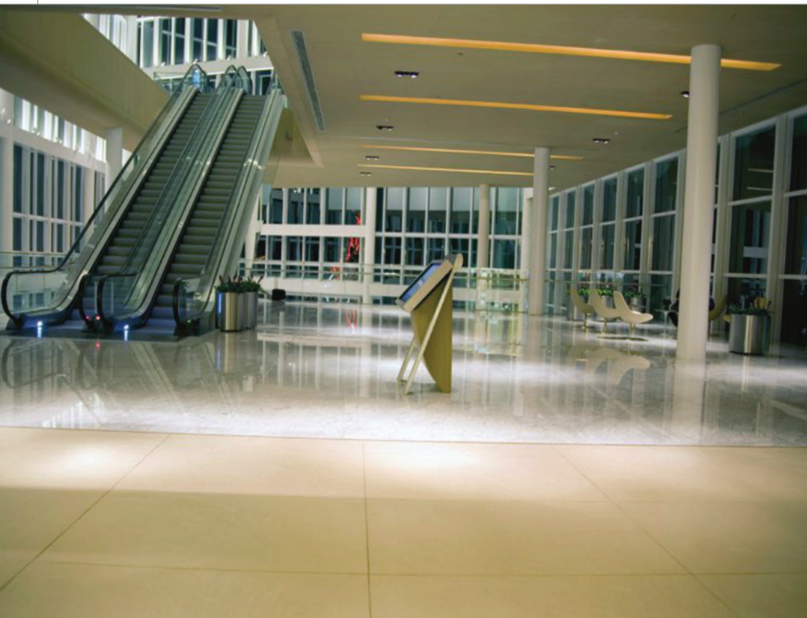
O piso do VillageMall combina o mármore Carrara Gioia e o quartzo Wave Cancun The VillageMall floor combines Carrara Gioia marble and Wave Cancun quartz
